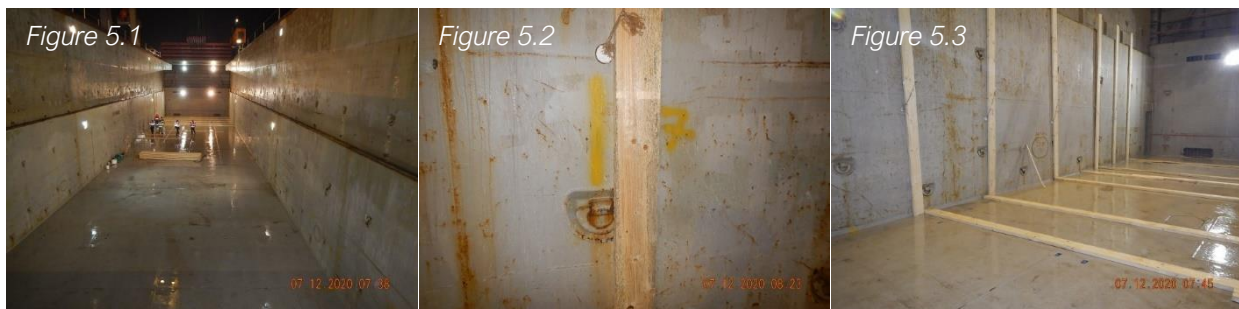
Dunnage Preparation – Pre-marked frame locations – Dunnage Bedding
