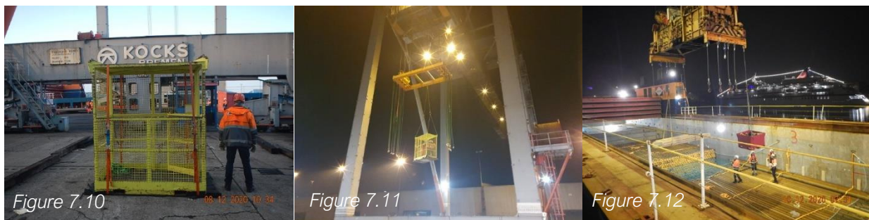
Personnel Cage – Cage Lift – Transfer of Dunnage and Tools
