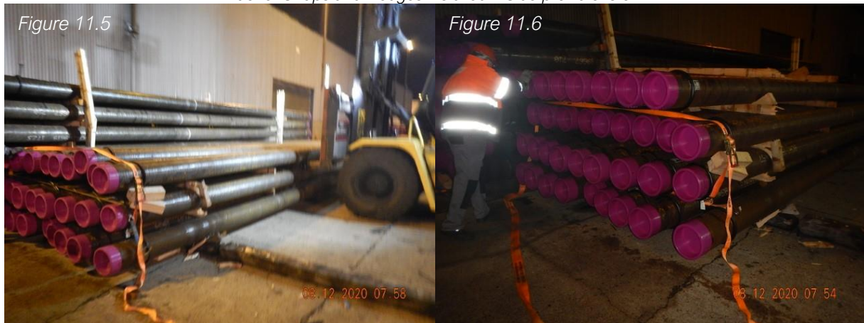
Tier by tier removal of remaining pipes
