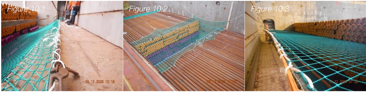
Installation of safety nets
