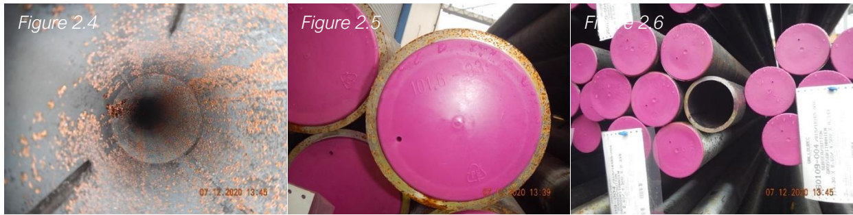
Internal condition – 101.6mm end caps fitted to 114.3mm pipes – Missing end caps
